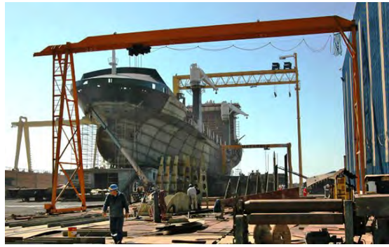
Aluminium Construction - Outdoor construction for larger vessels
